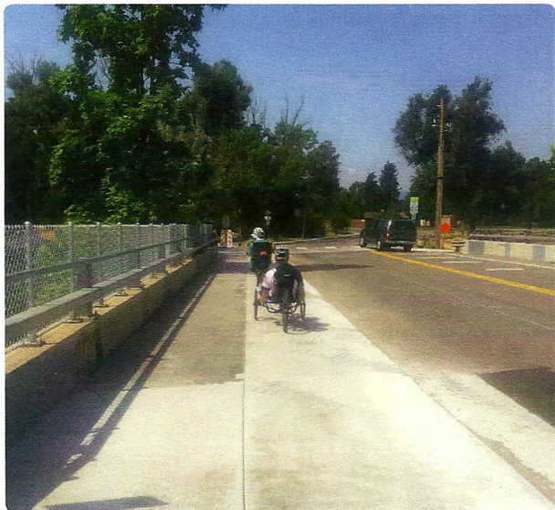
AFTER – Lowell Boulevard area
