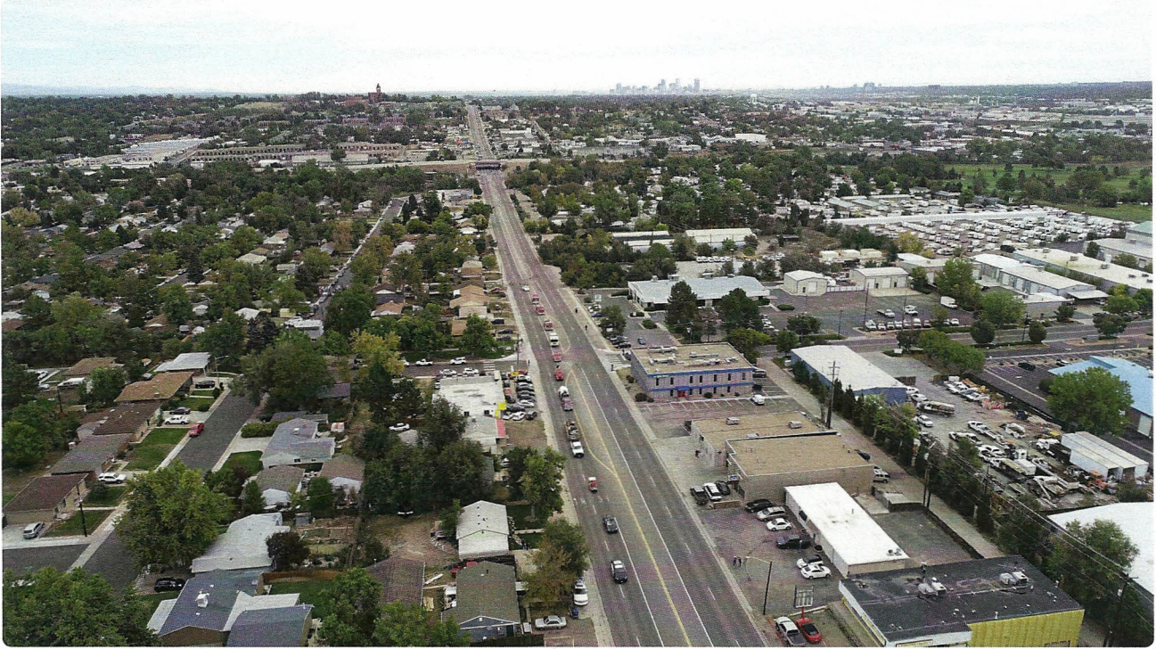
BEFORE – South Federal Boulevard
